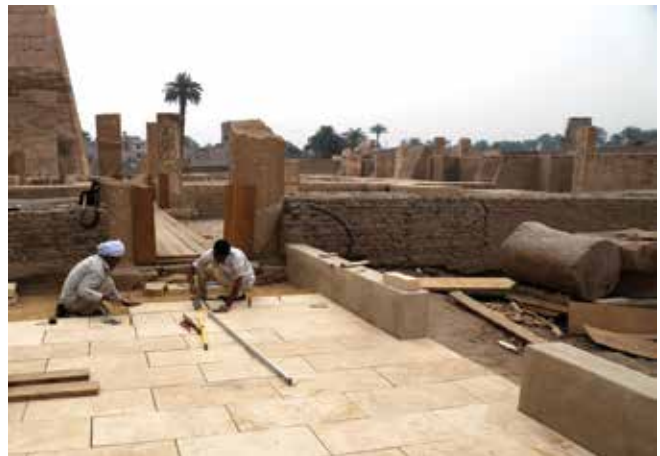
Finishing viewing platform flooring. Medinet Habu. Photo by Frank Helmholz
