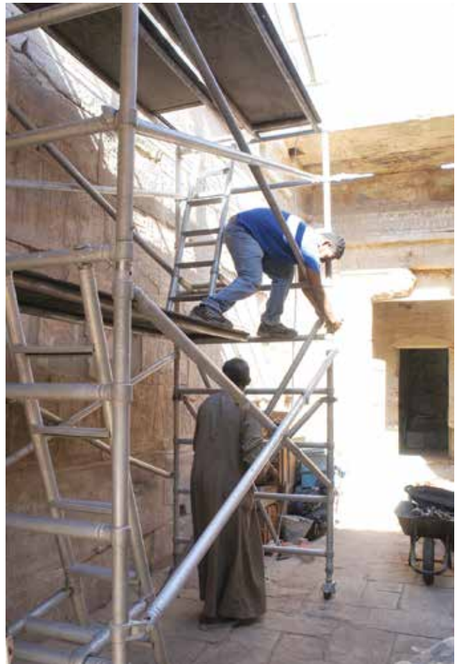
Setting up scaffolding in the small Amun temple. Medinet Habu. Photo by Ray Johnson
