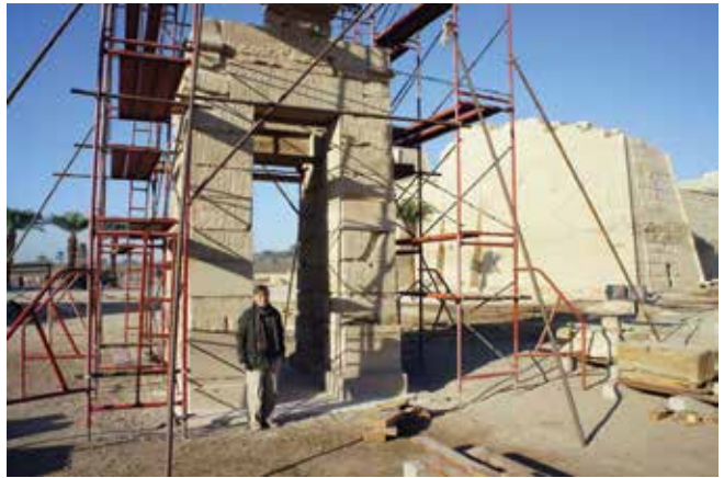
Frank and the completed Domitian Gate. Photo by Ray Johnson
