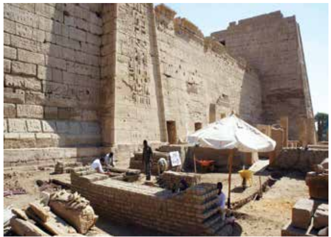
Capped brick walls and viewing platform underway. Medinet Habu. February 19. Photo by Ray Johnson
