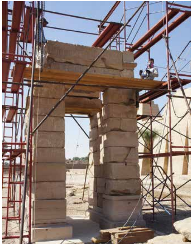
Johannes placing restoration stone. Domitian Gate, Medinet Habu. Photo by Ray Johnson
