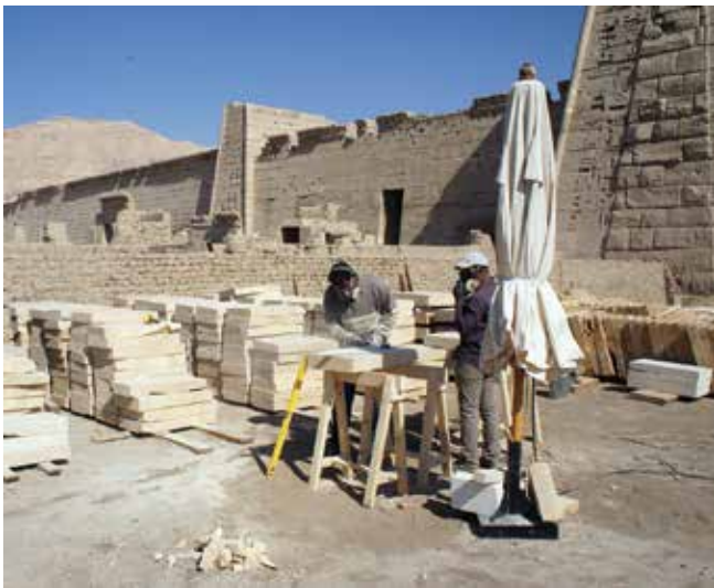
Mohamed and brother Mahmoud shaping sandstone slabs for the viewing area and walkway. Medinet Habu. Photo by Ray Johnson
