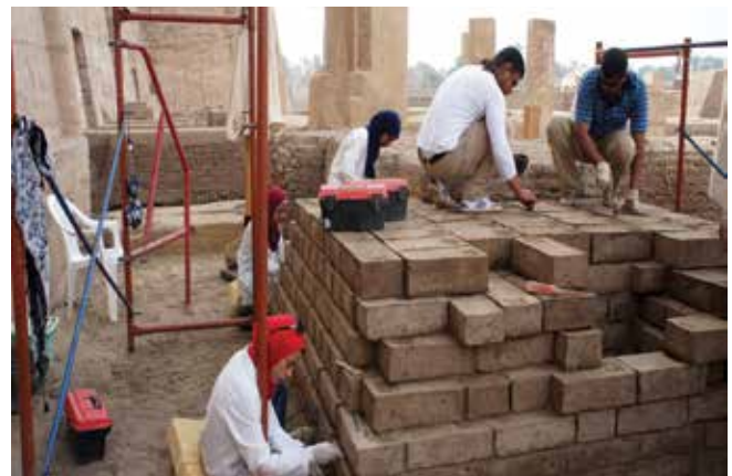
Brick-wall restoration going up. Medinet Habu. Photo by Ray Johnson
